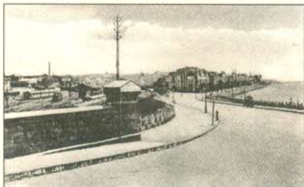
Colaba Reclamation from Wodehouse Bridge, Bombay Photograph given by Sharda Dwivedi
